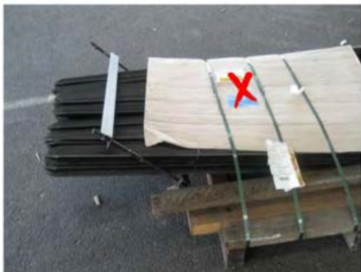
There has been no lateral restraint applied to these star pickets.
